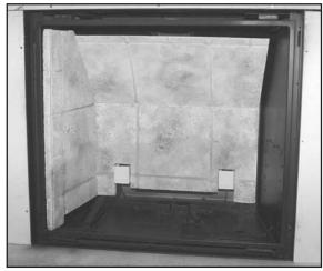
Figure 65: Top Firebox Liner Panel in Place.
