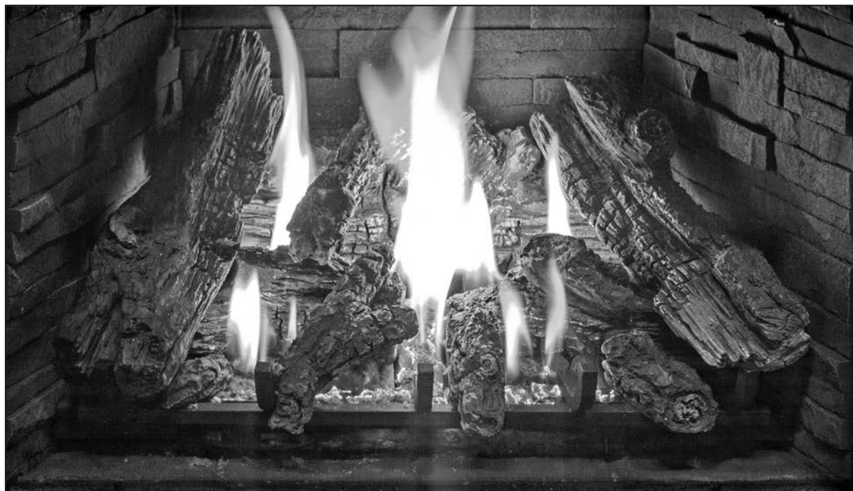
Figure 54: Proper installation and flame appearance
