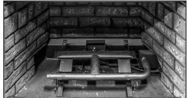
Figure 41: Remove the 6 screws highlighted in figure 40 using a Torx T-20 screwdriver and remove the air deflector
