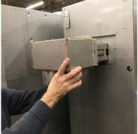
3. Push the gasketed surface of the heat exchanger up tight to the body of the fireplace and secure using the (10) screws removed in step 1.
