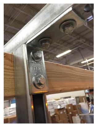
Run the 3/8" all-thread provided from the top piece of Unistrut® to the lower as shown in the pictures below. This will be used as fine height adjustment later. Bolt the 2 vertical members of Unistrut® to the lower piece using the  $1-5/8 \times \frac{1}{2}$ " channel connectors, bolts and washers provided.
