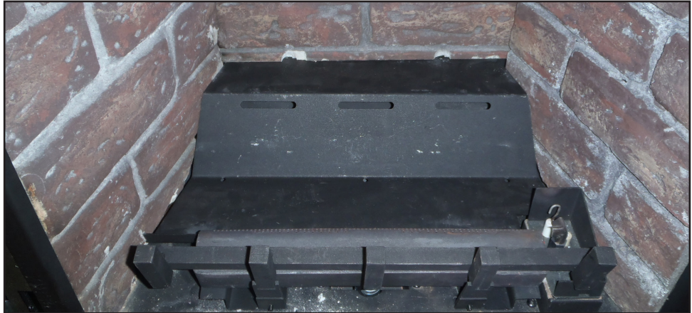
Figure 35. Empty firebox with grate and locator pins.
