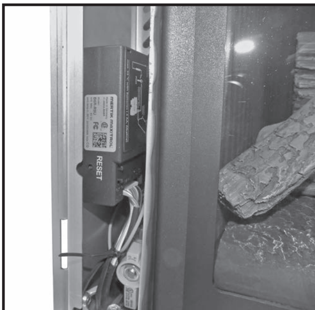
Figure 21: Maxitrol reset button location.
