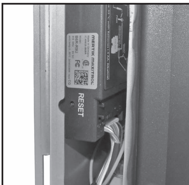
Figure 95: Maxitrol reset button location.
