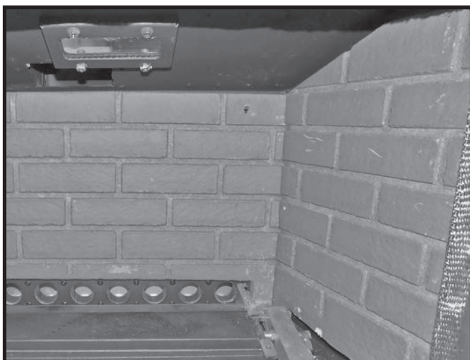
Figure 28: Right side panel in place.
