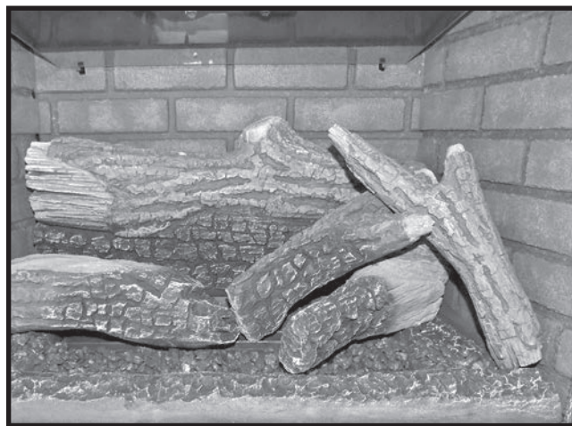
Figure 80: 5th log placement.
