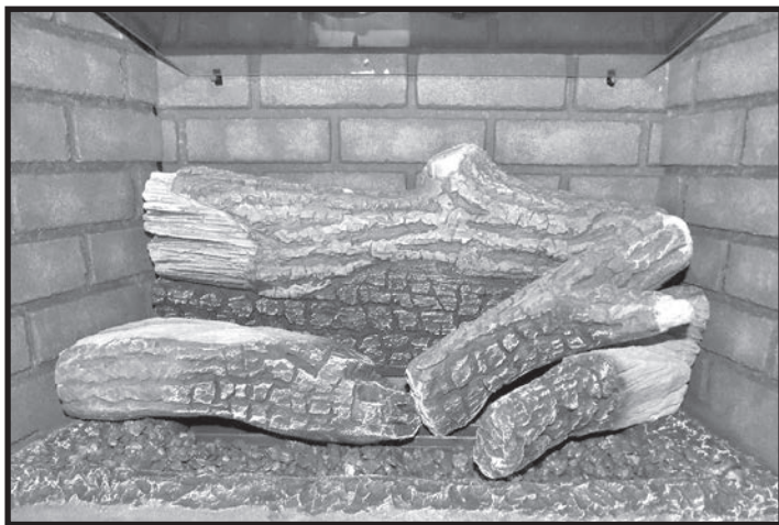
Figure 79: 4th log placement.
